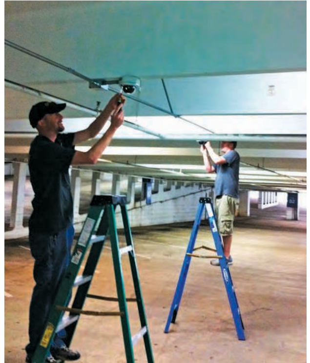
Ryan Armstrong (left), crew leader and Josh Davis, senior technician, work on camera and conduit installation after Dallas Galleria operating hours. While the initial intent was to minimize disruption to the shopping center, the off-hours work sped up installation dramatically as it presented a safe and obstacle-free environment that would have been difficult to achieve with heavy traffic in these areas.
