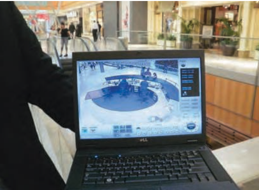
IP cameras are reviewed and focused using a laptop PC at the field device location. Here, cameras are installed in the Guest Reception Booth to add coverage and document activity.
