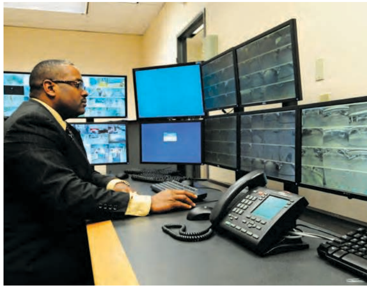
Galleria Dallas Director of Security Earl Morgan reviews camera coverage and field of view as devices are brought online. By not waiting for a final punch list, corrective action can be taken while the crew is still working in that area, reducing the number of return trips and speeding up the final testing and tuning.
