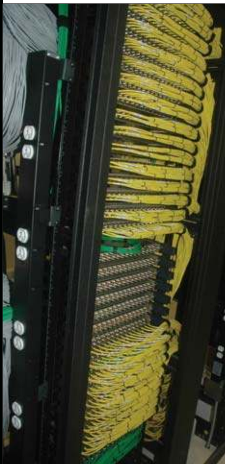
Analog matrix switching systems provide real-time switching and control with very little latency. Applications that do not require time-intensive camera control can utilize the virtual matrix.
