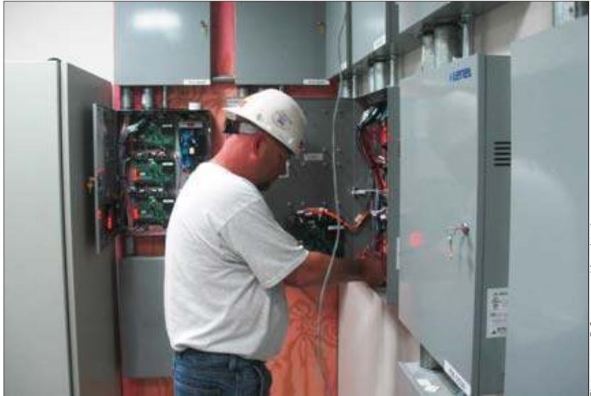
Photo courtesy R. Grossman and Associates Inc.
