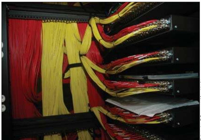
Unshielded twisted pair (UTP) signals are fed to Nitek active hubs to be converted back into unbalanced signals and transmitted to both the matrix switch and digital video encoders. Each hub provides two individual outputs per camera, allowing the systems to be fed separately (via color-coded cabling) and preventing a problem with one system impacting the other.
