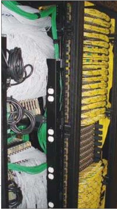
Photo courtesy R. Grossman and Associates Inc.
