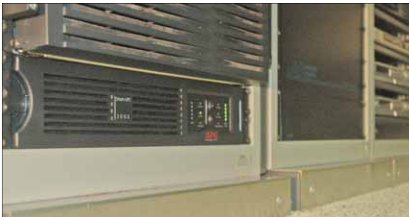
An uninterruptible power source (UPS) is deployed between a power supply and a device, such as computers, to protect equipment from the adverse effects of power outages, sags, surges and the like. A centralized UPS or standalone device, such as the APC 3000 Series unit pictured above, is an essential part of the foundation of every security system.
