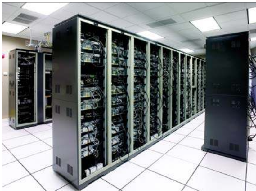
Since digital video servers and RAID storage vents from front to back, vertical racks in the new rack room were left open to improve air flow and avoid heat pockets, which can reduce the lifespan of hard drives.
