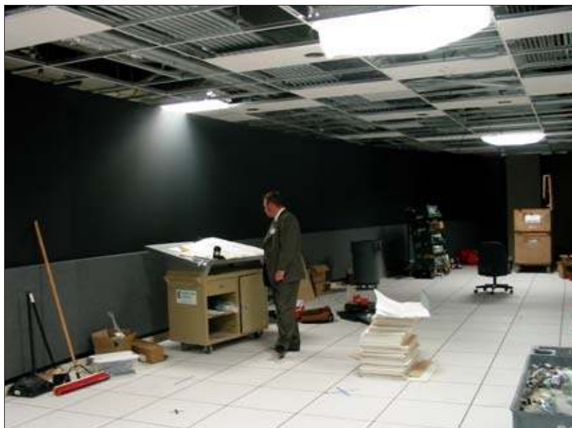
Surveillance Director Richard Thake surveys the control room plans before the arrival of the console and video screens. The gray fabric components on the lower portion of the video wall are acoustical panels that dramatically reduced sound reflection, making the room quieter and more comfortable for long shifts.
