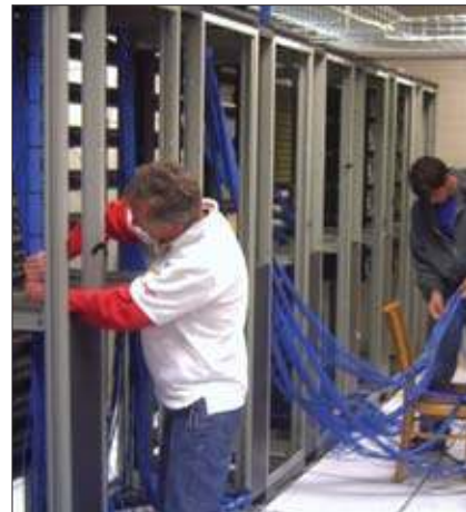
Data cables are pulled from the digital video encoders to the patch panels.
