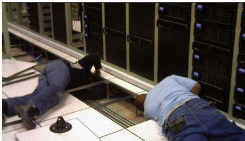
A raised computer floor was used in the rack room and control room.
