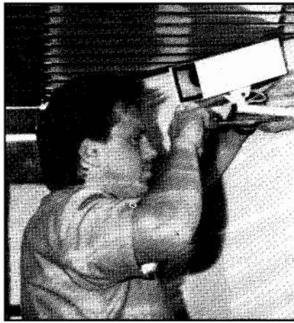
Decorative camera housings were used on the skywalk People Mover.
